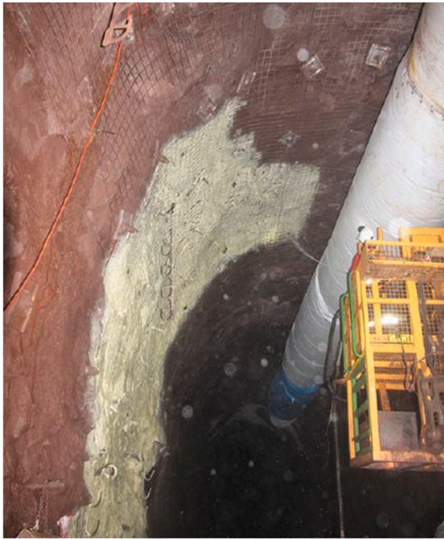
Fig. 37. TSL provides a protective barrier for the mesh and bolts in the Carrapateena mine. Taken from [188].
